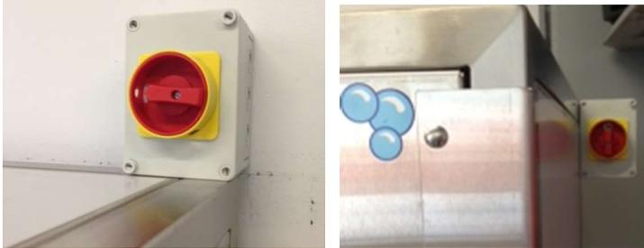
Shown on the right is the main electrical cable inside the dog wash. It enters through the gland at the bottom of the dogwash close to the ground. Run the power cable in 25mm flexible conduit as there is a socket already installed into the bottom of the main circuit breaker box shown. Leave 1m in length after you have reached the bottom gland.
