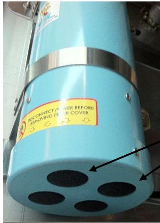
This picture highlights the 4 foam filters located at the base of the dryer that requiring cleaning
